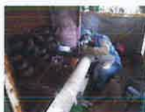
Modifying convection coils
